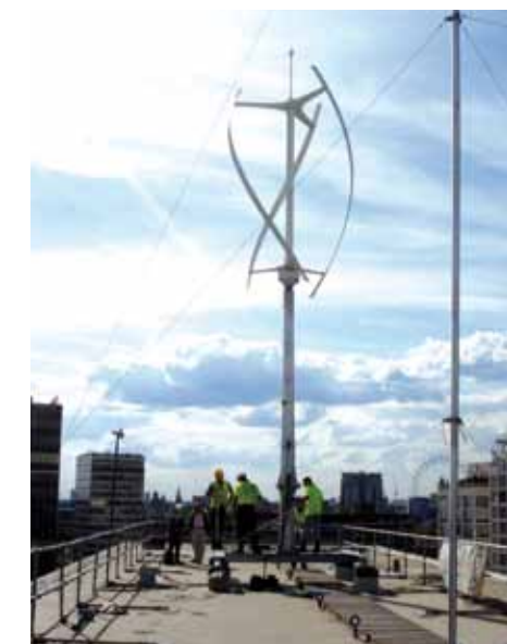
Ground mounted wind turbine installation
