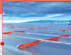
Pelamis offshore Wave Farm
