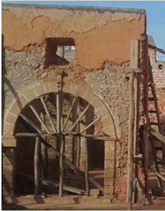
Figure 2. Restoration works inside the barrack
