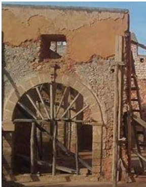
Figure 2. Restoration works inside the barrack
