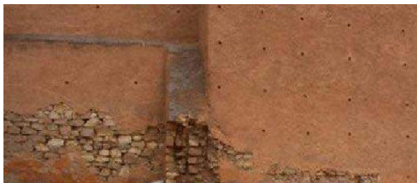
Figure 3. Two years after restoration
