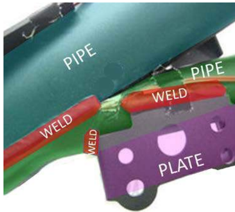
Figure 3. Pipes and plates welded together to form the frame.
