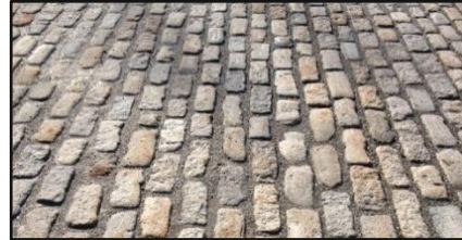
Image of Belgian block surface [3]
