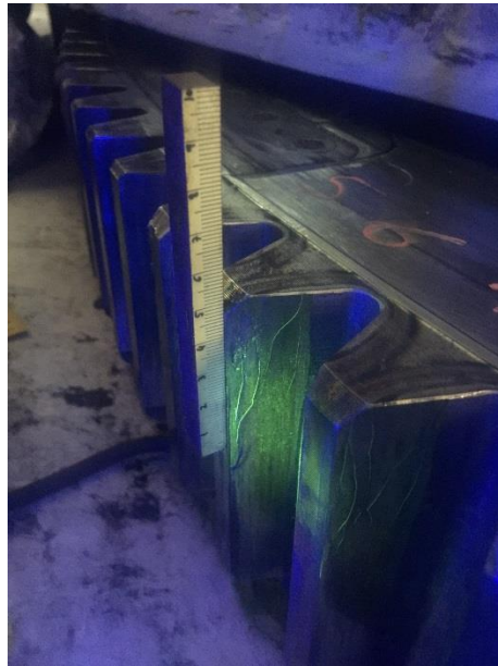
Figure 9. View of representative cracks.
