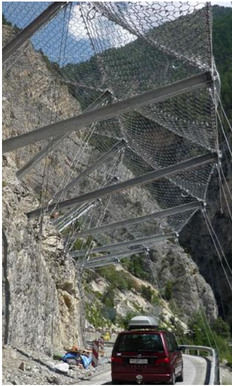
(a) Rockfall canopy
