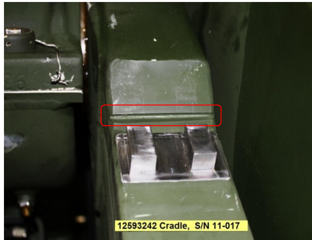
Figure 1. Rear Cradle Structure with Groove Highlighted in Red.
