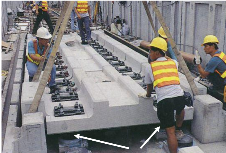
Figure1. Installation of floating slab track for Hong Kong Airport rail link. Arrows show location of rubber bearings. (From www.urbantransport-technology.com/projects/hong_kong )
