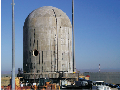
Figure 1: 1:4 scale PCCV prototype (Ref. 1).
