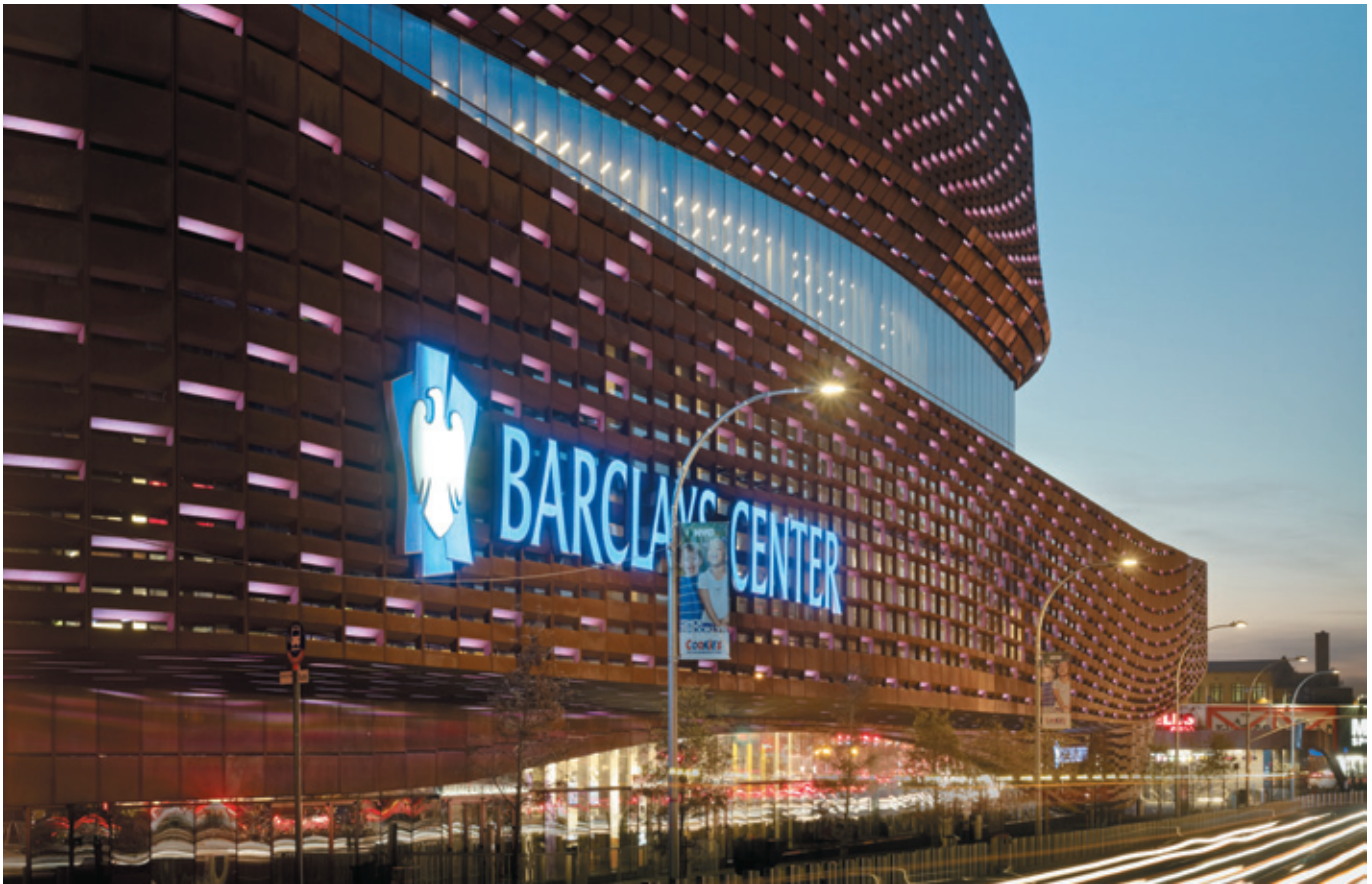
The facade of the Barclays Center features 12,000 pre-weathered steel panels, each different in size and curvature. The 3DEXPERIENCE Platform and CATIA application were instrumental in managing the resulting complexity of design, fabrication and installation. (Photo here and on cover by Bruce Damonte)
